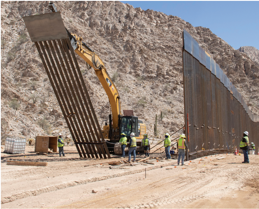
U.S. Army Corps of Engineers South Pacific Border District contractor crews place barrier panel along the U.S.-Mexico border near Yuma, Arizona. (Photo: Orville Collins)
