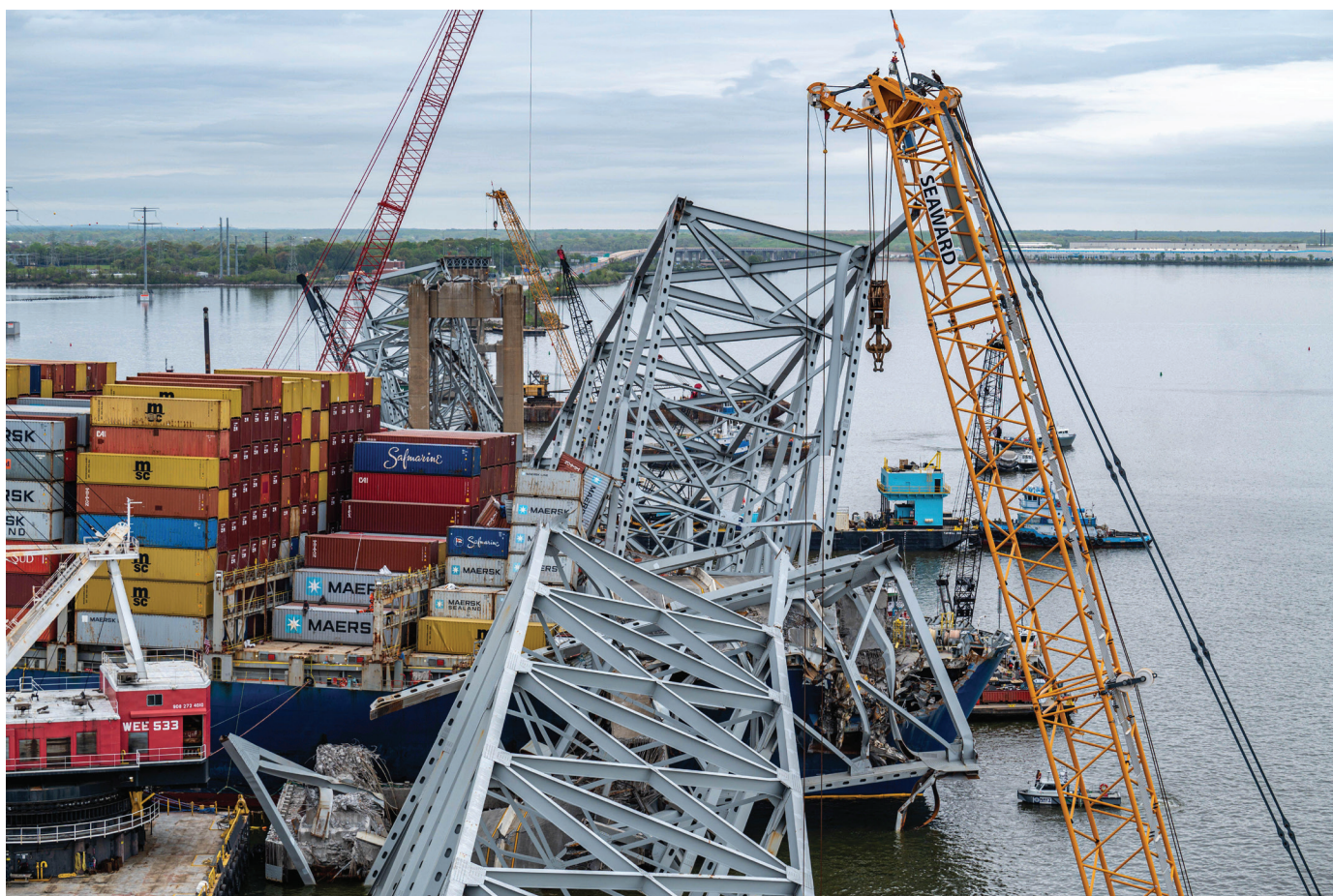
Crane barges lift wreckage of the collapsed Francis Scott Key Bridge from the MV Dali container ship in the Fort McHenry channel in Maryland. (Photo: MC2 Theodore Lee / US Navy)
